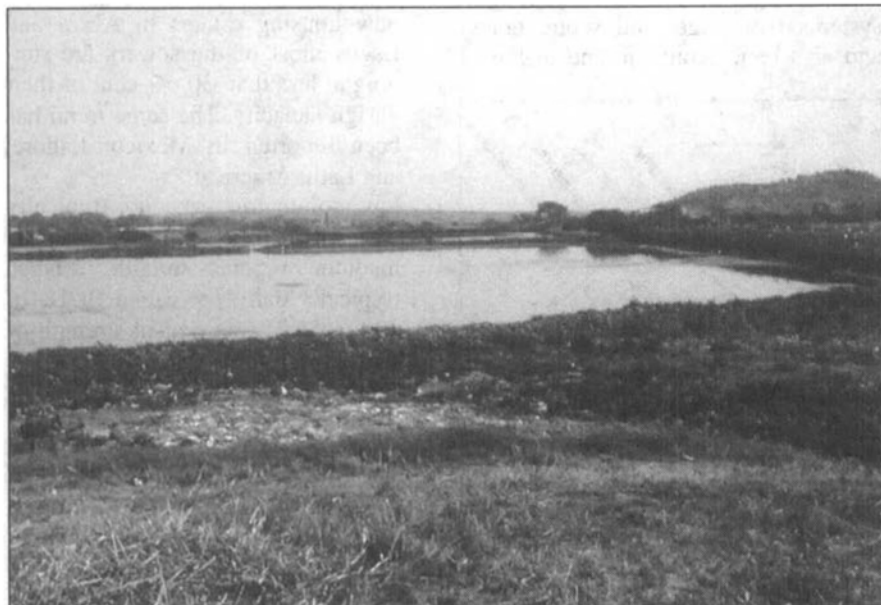
Simpler wastewater-treatment technologies — such as this waste-stabilization pond in Lusaka — are proving to be as effective as conventional plants.
