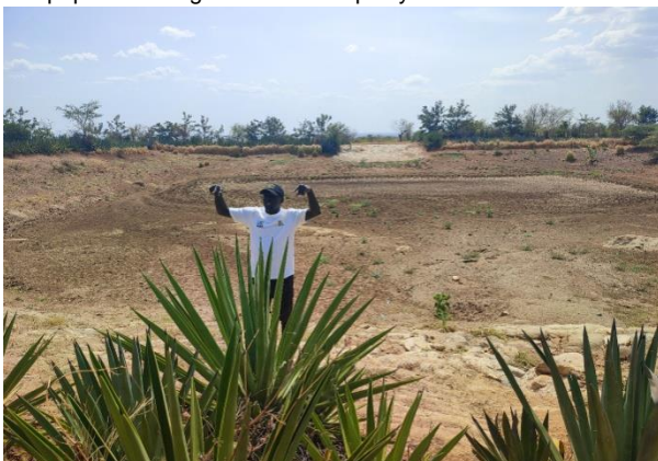
Figure 14: The valley tank was found empty because it had dried up
