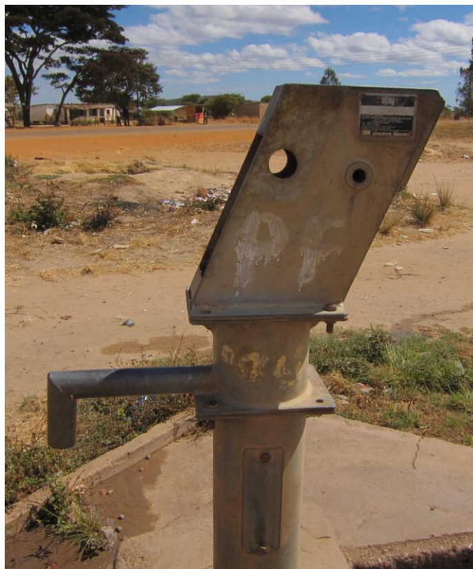
Broken down India Mark II handpump in Zambia
