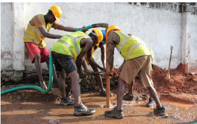
Figure 2: Drill Crew undertaking well jetting in Nigeria
