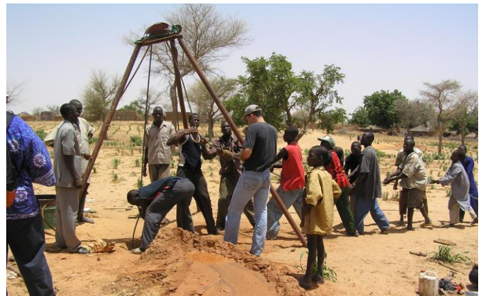
Figure 3: Percussion Drilling in Niger (Source: Richard Carter)
