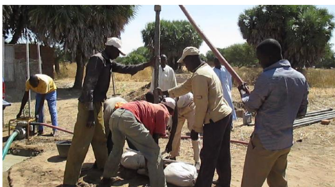
Figure 13: Jetting a household supply in Clesoum, N’Djamena
