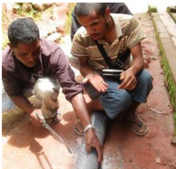
Figure 9: Masons cut slots in casing in Madagascar
