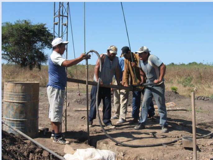
Figure (above) EMAS Percussion-Jetting-Rotation manual drilling, Trinidad, Beni region (Source Mike MacCarthy)
