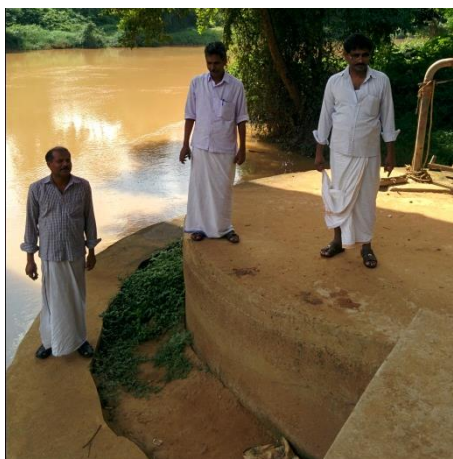
Photograph 7: Beneficiary Group members in front of Infiltration Tank of Cheruparambu Scheme
