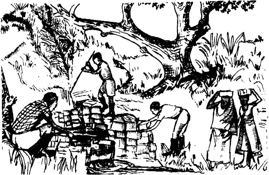
Fig. 8.5 Protecting a spring.
