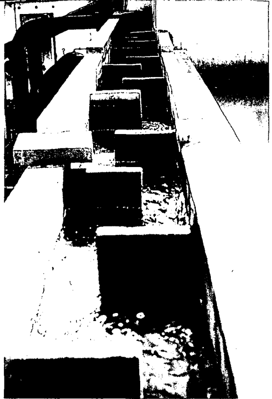
A properly-designed baffle flocculator of this type can provide a good treatment with little to go wrong.
