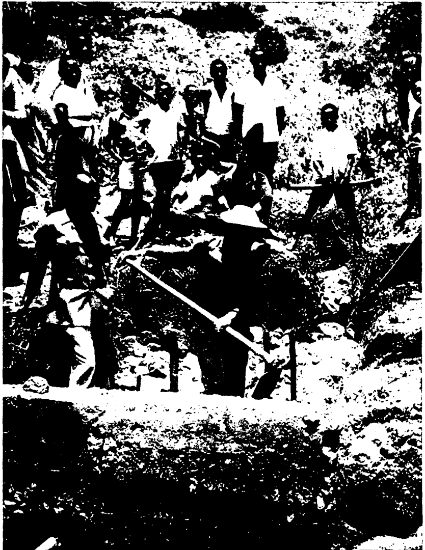
Construction work in progress at a spring site.
