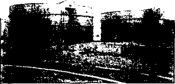
Drinking water storage for ships' bunkering in the Far East. Total capacity 726,000 litres.
