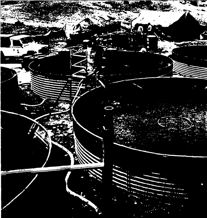
OXFAM emergency water treatment plant
