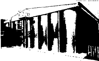
445,500-litre aluminium Liquitainer for a fire protection system.
