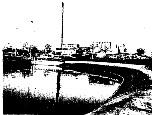
Biological waste water treatment plant. Surface 5.120 m 2
