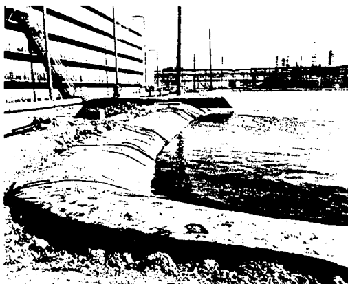
Holding pond of fresh water for treatment of oil and brine. Surface 11.000 m 2
