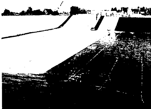
To contain process effluent in the event of break down of biological treatment unit. Surface 3.600 m 2
