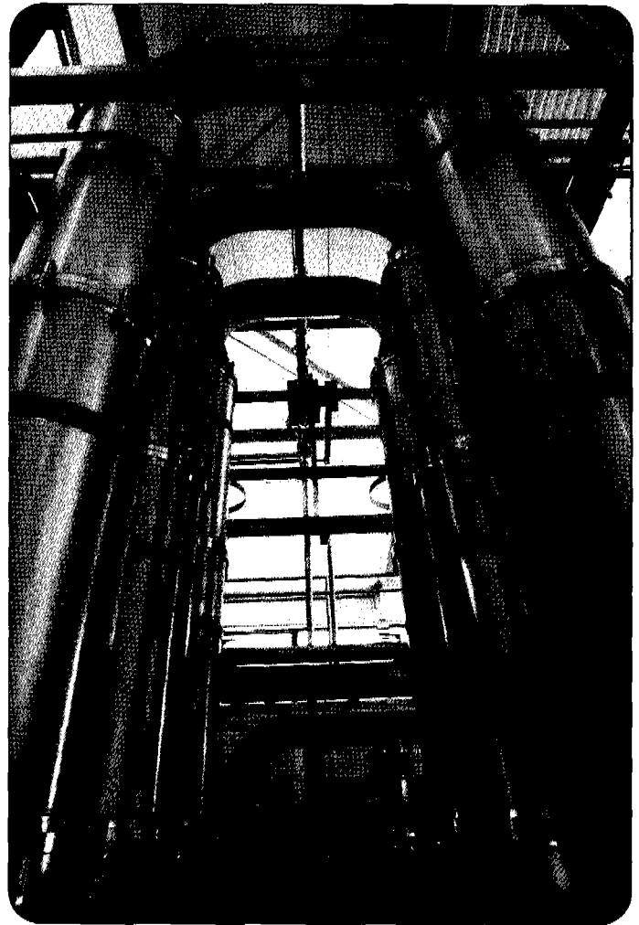
The Membrane Bioreactor (BRM) is used to treat industrial effluent and to produce water that can be directly reused
