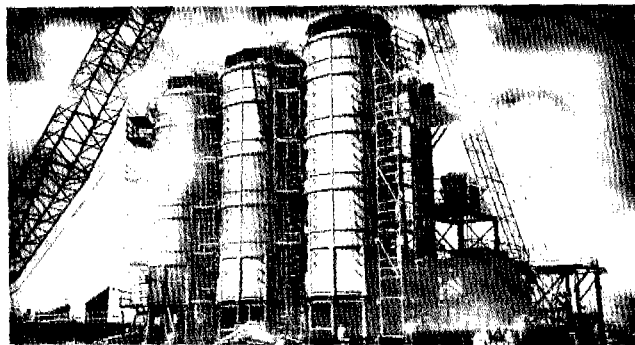
SEGHERSsludge Dryer & Pelletizer, Baltimore USA. Evaporation capacity 18.000 kg H 2 O/h. One of the largest sludge dryer & pelletizer plants in the world.
