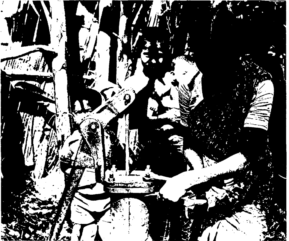
Fig.2. Participation of women in local maintenance: a woman caretaker using a wrangle to repair one of the many no. 6 hand pumps in Bangladesh (IRC photo by Akil Khan).
