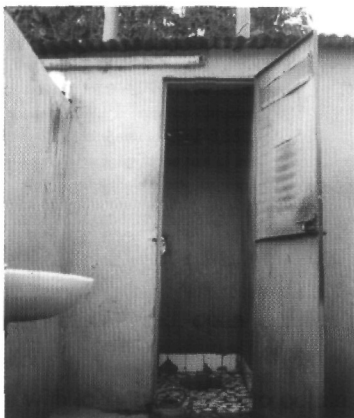
VIP latrines and showers in small neighborhood markets, as envisaged by the Strategic Sanitation Plan for Bamako.
