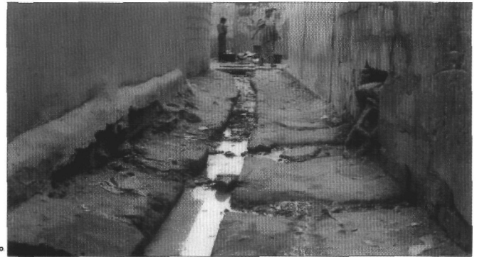
The sewerage network is very limited in Bamako
