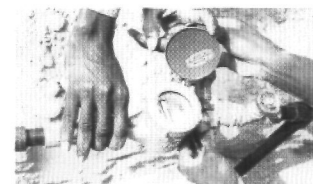
Network extension works and installing house connections.
