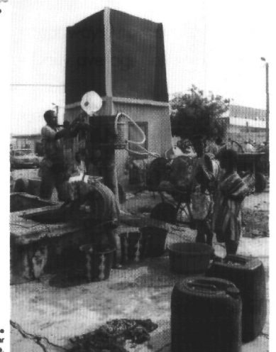
An improved standpipe model located near a conventional one.
