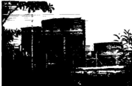
In this clarifying basin sedimentation does not take place at the bottom of the tank.
