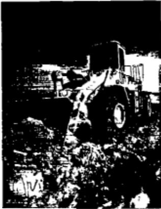
*Spreading and compacting solid wastes at a landfill site*
