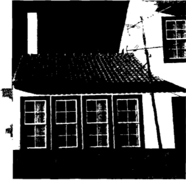
Above: A wing of a new school being constructed as part of a large educational complex for retarded children in Guarda. Guarda's MERECE design team introduced design alterations that led to incorporation of locally quarried granite and locally harvested wood into the building. The school also features wood window frames, wall insulation, insulated storm shutters, wood stove heating, and other MERECE principles
