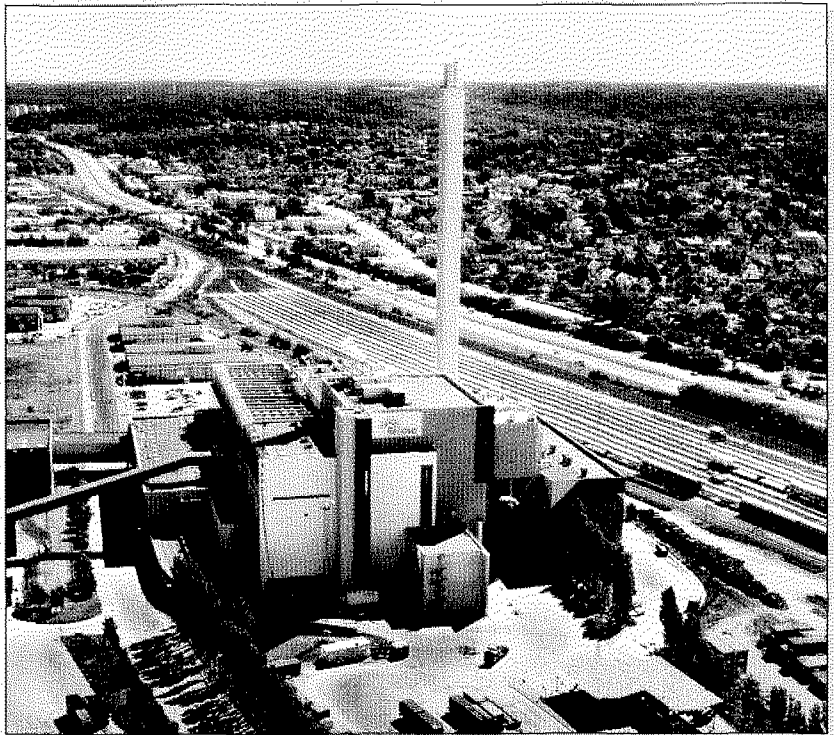
Figure 4 Incinerator of solid waste
