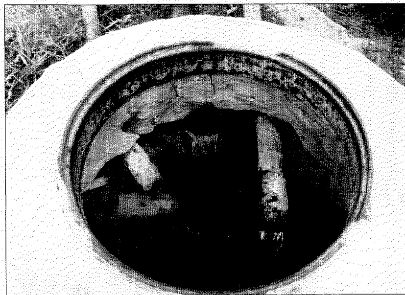
Figure 4 Rusting and disintegrating pipes
