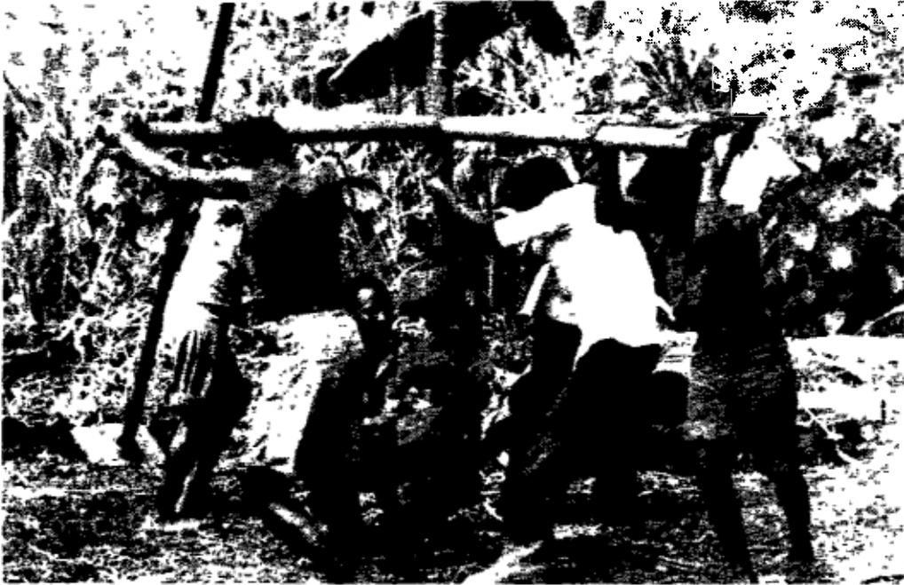
Figure 8-12. Hand drilling in operation in Morogoro.
