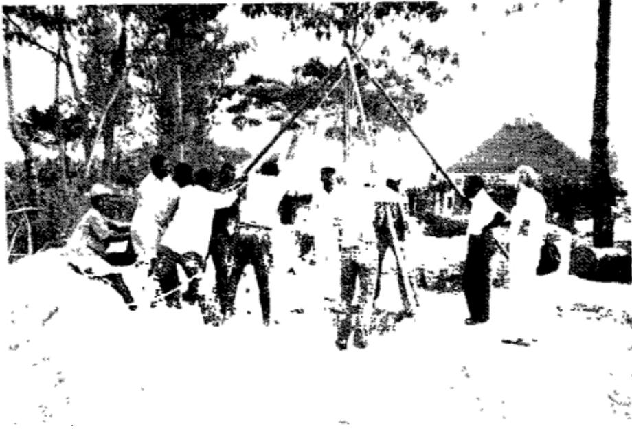
Figure 8-7. The well ring installation by using a tripod.
