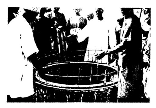
f) Pour concrete into mold until full. Tamp down the cement with long sticks as it is filling to eliminate air bubbles. Smooth top of buse. Make sure loops are centered.
