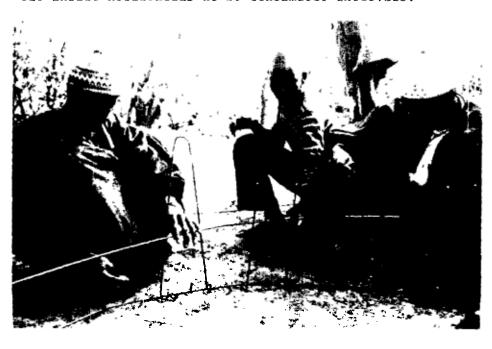
c) Horizontals should be spaced at an even distance from each other. Make sure the assembled cage will fit entirely into the buse mold. Bend 4 longer pieces of rerod with hooks at the bottom and tie them onto the outside of the horizontals, evenly spaced. These loops will extend over the top of the buse mold and will later be used to tie the rope around for lowering them into the well.
