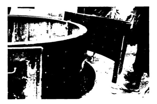
e) After pouring wet concrete into bottom 5 centimeters of the mold, lower the assembled rerod cage inside.
