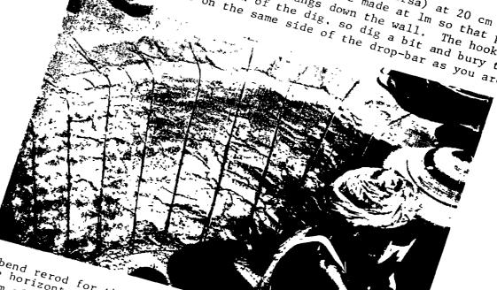
Cut and bend rerod for the place the horizontals (circumference plus 30 - 35 cm).
