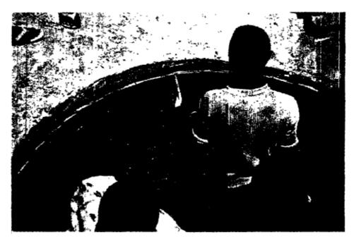
5) Prepare a 4 to 1 water/cement mixture. Mix it well and splash it onto the well wall and the lip of the hole. This mixture helps seal the wall, prevents crumbling into loose sand, and gives the plaster an adhesive receiving surface.
