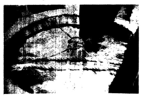
The rope used to lower the casing should be securely tied around the intersection of these two pieces of rerod.
