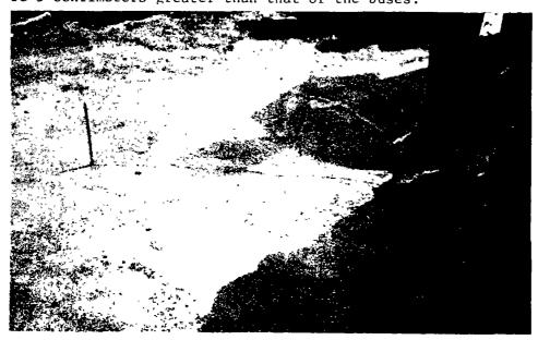
b) Using a wooden model as your guide, trace out the correct shape in the hole after you have dug it out roughly to size.
