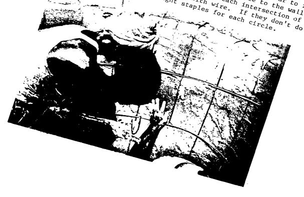
10) Apply the second coat of plaster but start 15 cm from the bottom of the dig. Smooth and plumb the wall with a trowel or straight edge. Fill in all gaps.
