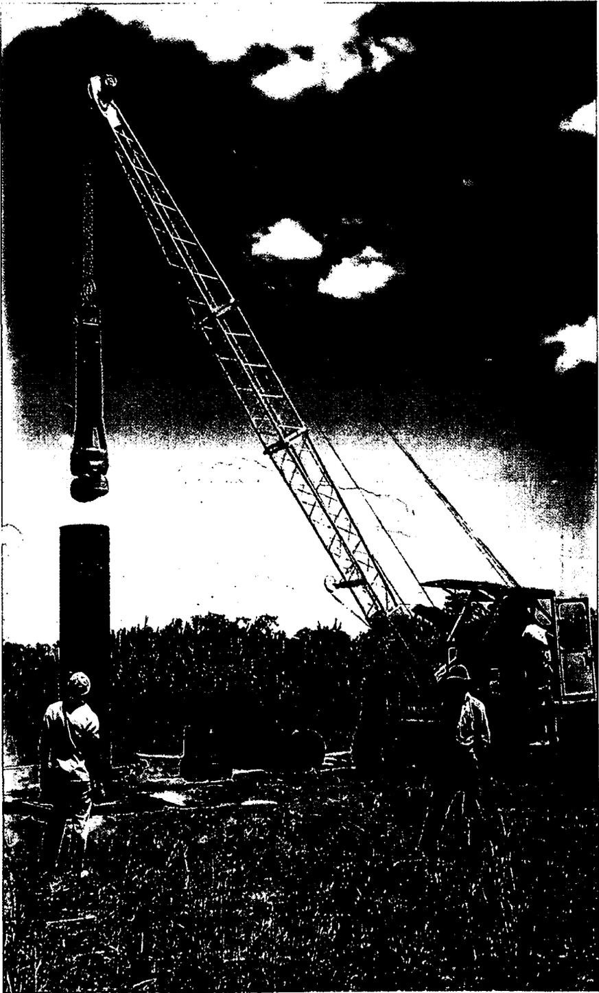
79. Mechanical well digging with clam shell
