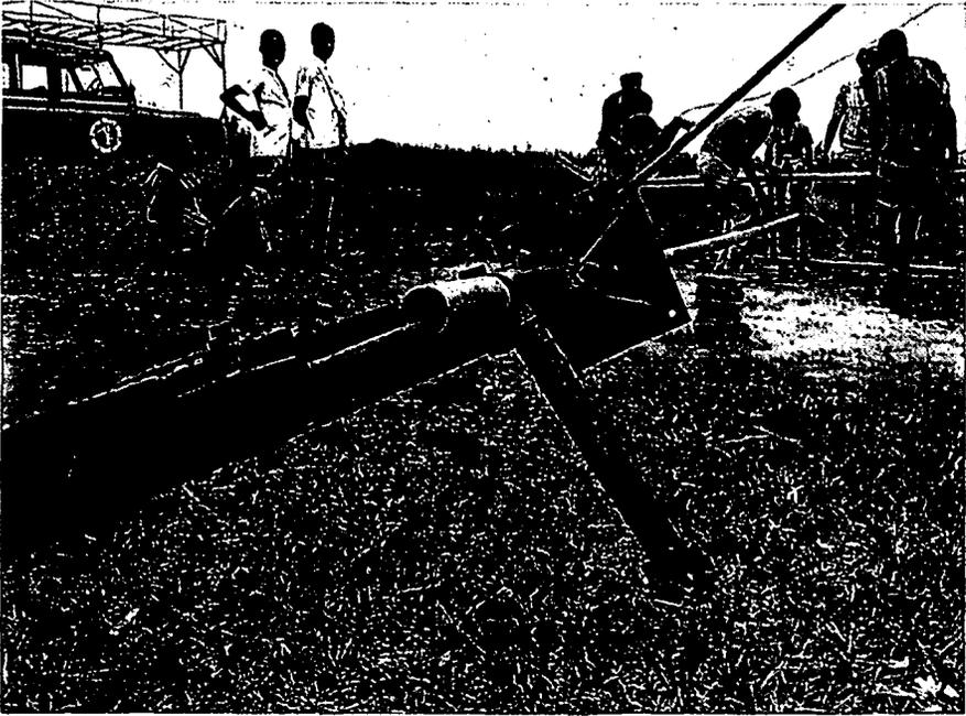
40. Single-acting hand pump. In background frame for positioning pump over well opening is visible
