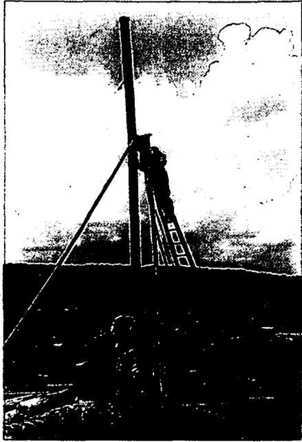
*72. The filter pipe is lowered in the borehole*
