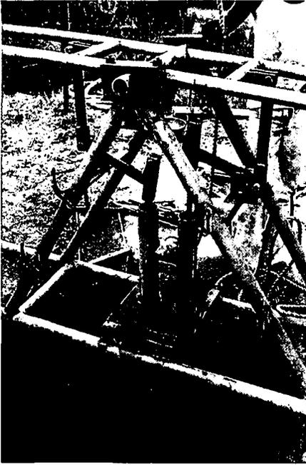
42. Double-acting hand pump, used during construction of wells (detail of superstructure)
