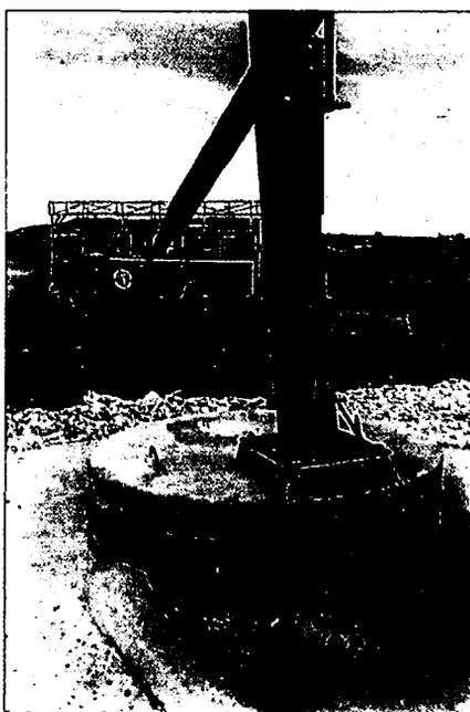
84. Detail of well superstructure. Note horizontal platform for buckets
