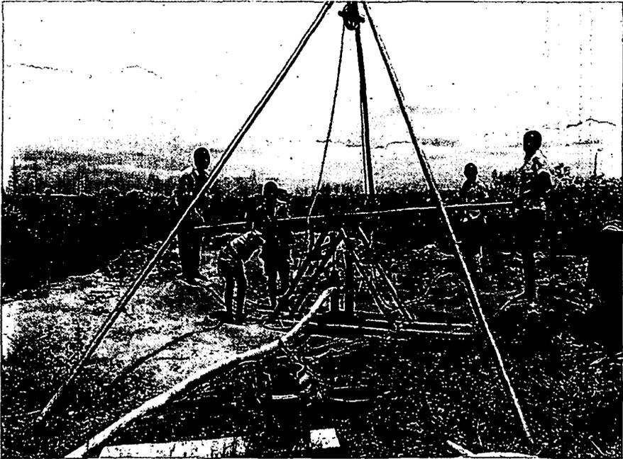
41. Double-acting hand pump, according to principle of old-fashioned fire-fighting hand pump
