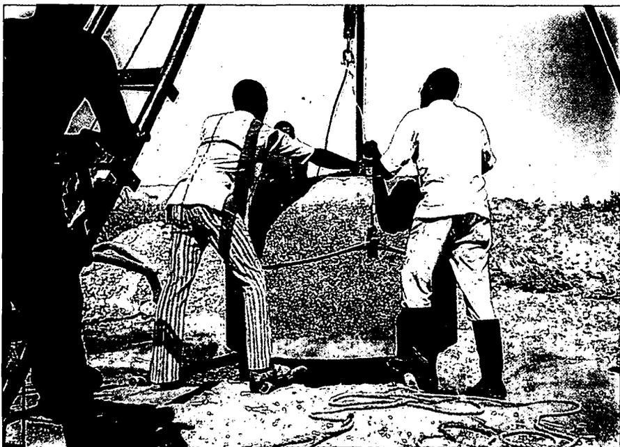
51. The guide-rope around the ring is repositioned to prevent askew lowering
