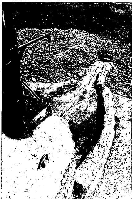
83. A gutter guides the spoil water to a drainage area
