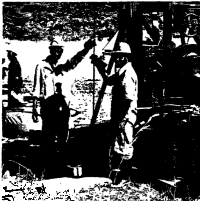
Figure 3.4 Cable-tool drilling in Zimbabwe
