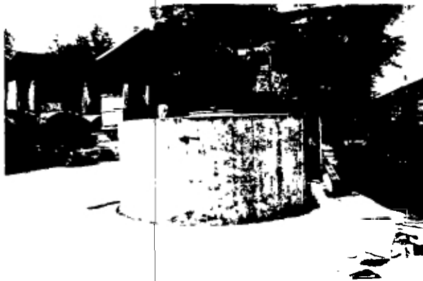
Fig. 16 Completed Tank B
