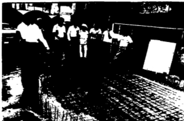
Fig. 7 Assembled Reinforcement for the Base
