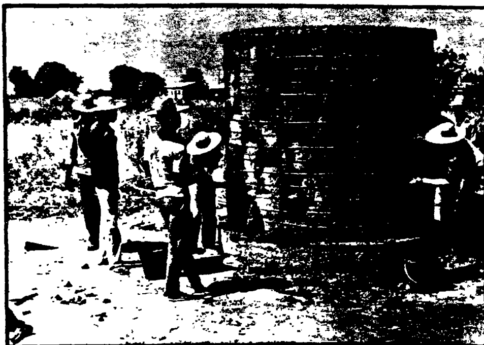
Photo . Trainees beginning to apply the exterior layer of mortar to the cistern.
