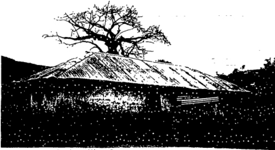
Photograph 2 Roof as a Water Source.
