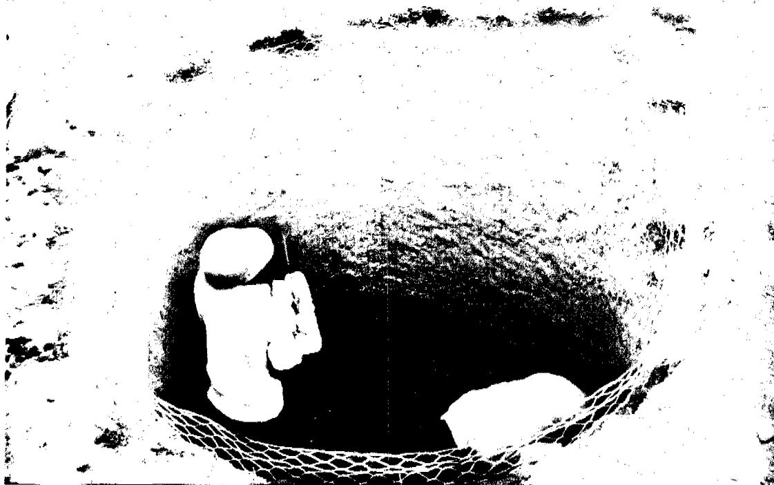
This tank was initially built for storage of water for construction during a training course at Kibwezi in Kenya in 1997. Upon completion of the training, the tank was equipped with a silt trap and used for harvesting water from a road.
