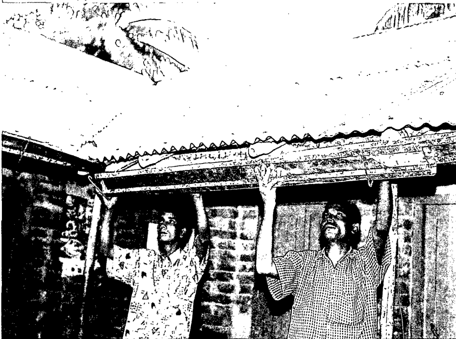
Hanger & Gutter Setting
