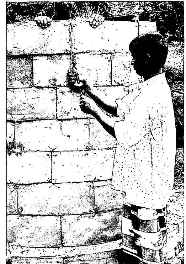
Setting of Cement Segments
