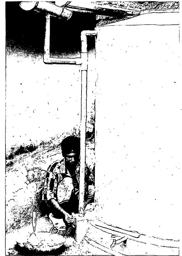
Flushing System & Storage indicator
