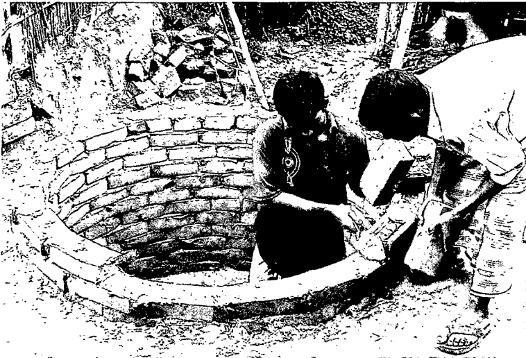
Construction of Brick Wall
