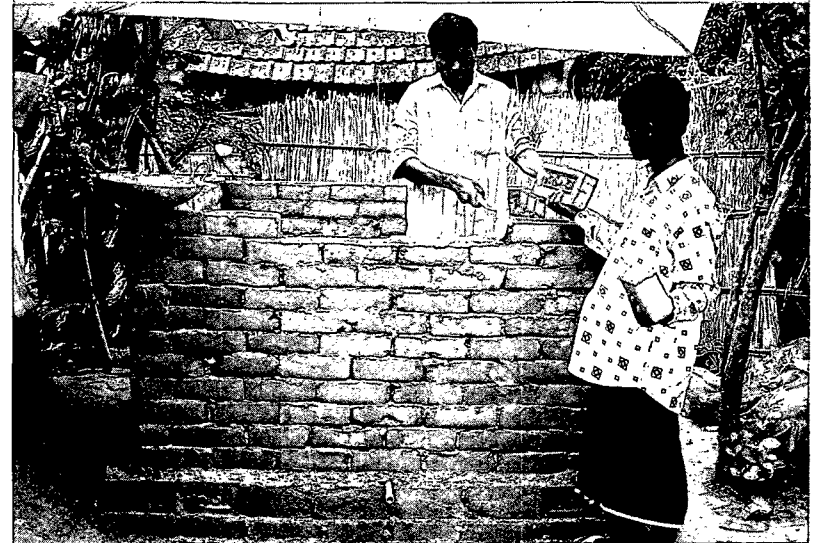
Brick Work on Tank Body
