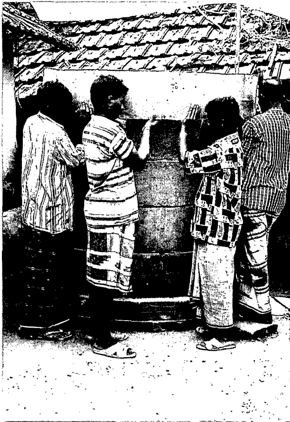
Setting RCC Ring
