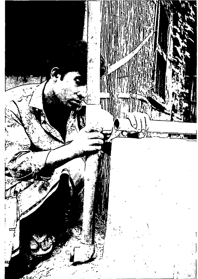
Setting of Flushing System
