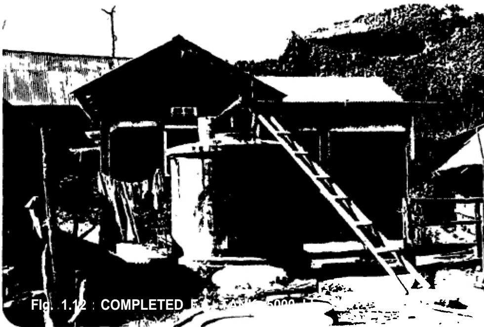
Fig. 1.12 : COMPLETED F.C. TANK, 5000 LITRE IN MARAN HILLS IN MANIPUR - FILTER BEING INSTALLED
