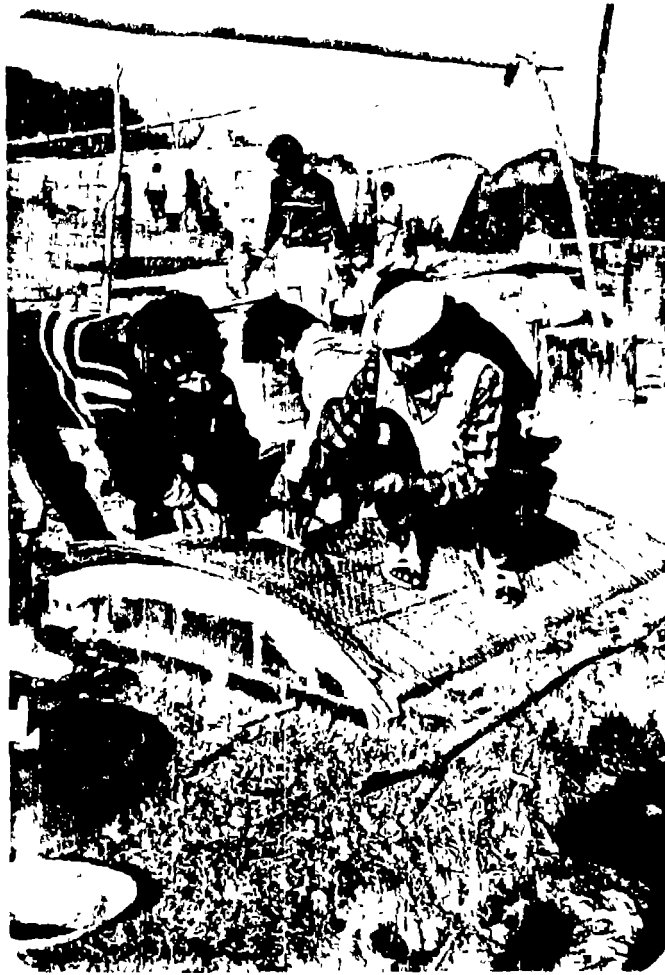
Fig. 3.3 : CAGE MAKING FOR A SEGMENT
