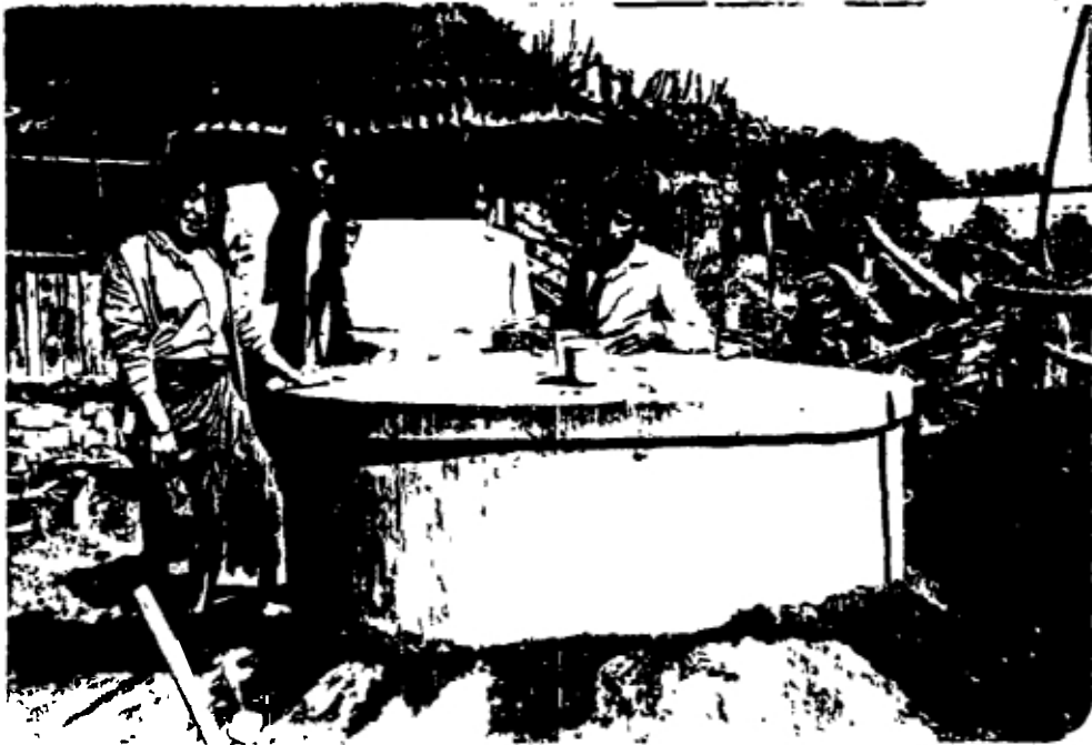
Fig. 1.11 : COMPLETED RAINWATER HARVESTING TANK 5000 LITRE - PARTLY ABOVE GROUND
