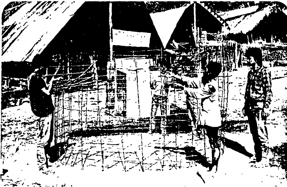
Fig. 1.8 : TYING OF WALL REINFORCEMENT CAGE
