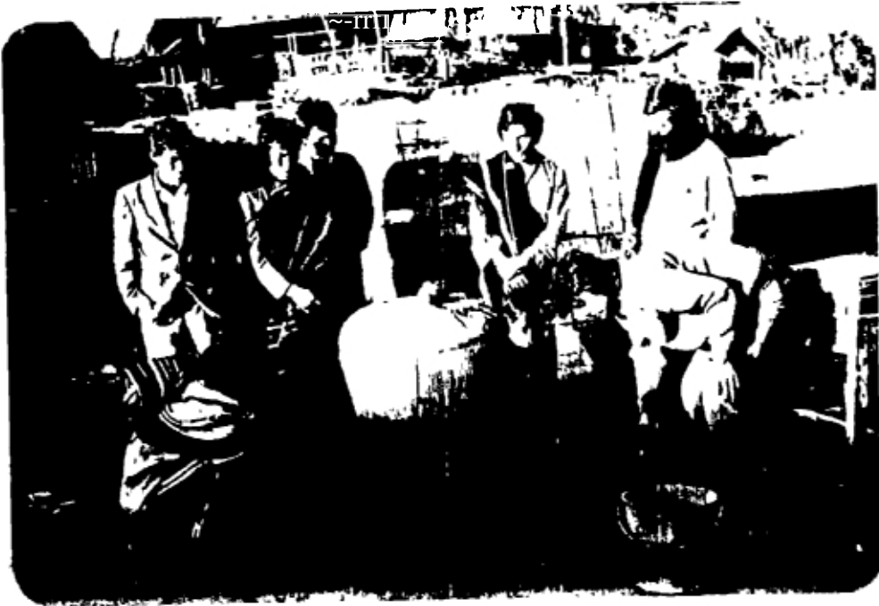
Fig. 6.6 : SACK MOULD IS FILLED WITH RICE HUSK - TOP CLOSED REINF. FIXED OVER THE MOULD
