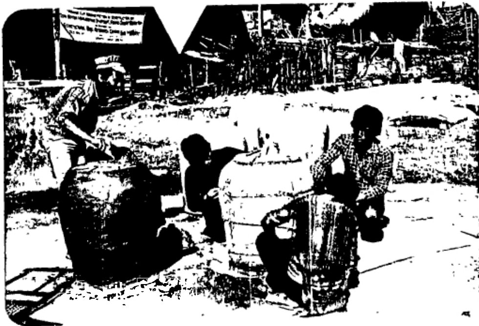
Fig. 6.7 : CASTING OF TANK BEING CARRIED OUT BY NAGA BOYS
