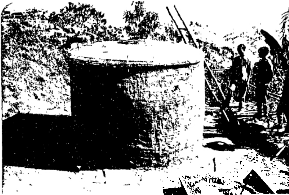
Fig. 1.10 : MORTAR APPLICATION FOR WALL & BASE COMPLETED THE CASE FOR ROOF PLACED IN POSITION
