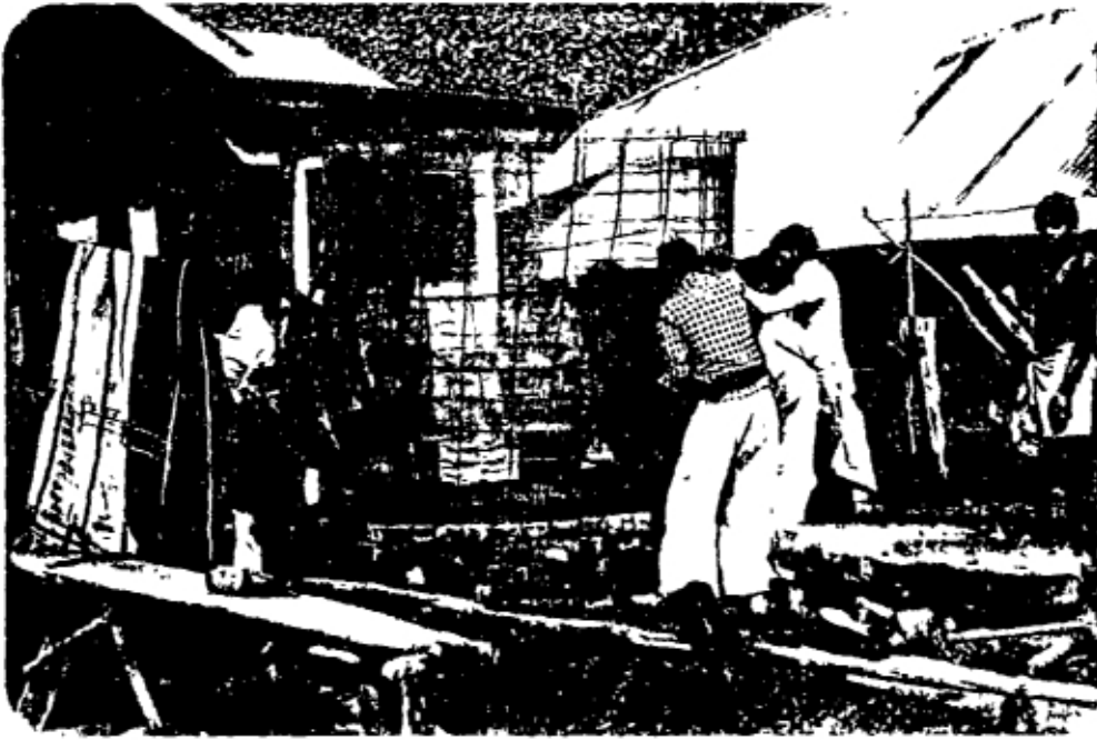
Fig. 1.9 : PLACING OF A COMPLETED CAGE IN POSITION — CAPACITY OF TANK 5000 LIT. LOCATION MARAM (MANIPUR)
