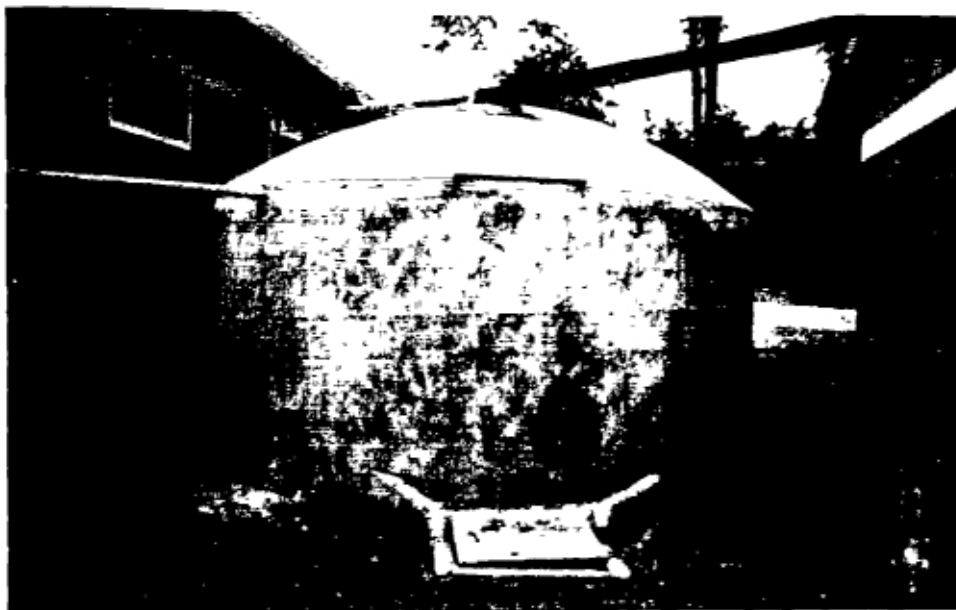
A 23 cubic metre water tank
