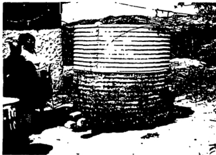
figure 2. the second wallring being constructed.
