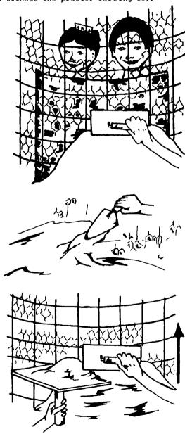
5. Plaster the outside of the tank in the same way as the inside. Leave for a day and water it to keep the tank wet and help "cure" the mortar.
