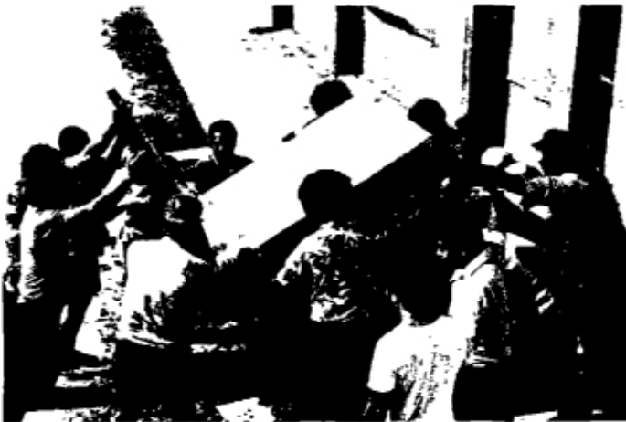
Illustrations 31 and 32: After three days, the tank is turned over on a pallet for convenient transportation to the site for utilization.
