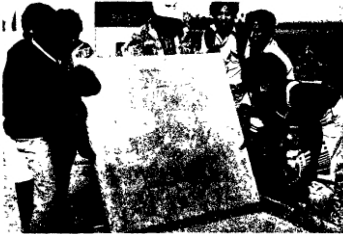
Illustration 20: Install the first vertical panel into position, pressed against the side of the box.
