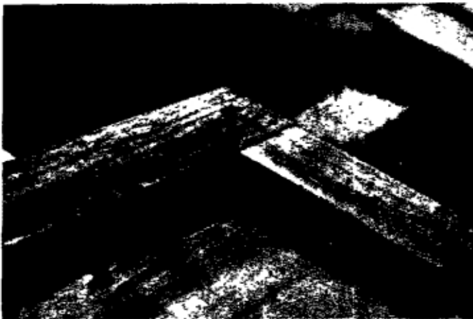
Illustration 13: The spacing bars are kept in position only by a single nail for each corner threaded through a hole provided at the end of each bar (Fig 1.6)
