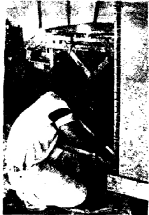
Illustration 25: The tamping rod is used to place and compact the mortar between the fingering wires
