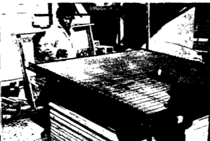
Illustration 42: The next layer is placed in the opposite direction in the spacing bar slots.
