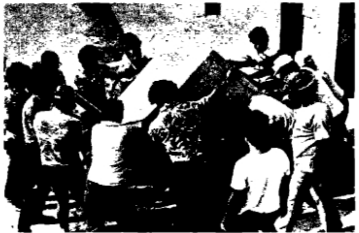
Illustrations 31 and 32: After three days, the tank is turned over on a pallet for convenient transportation to the site for utilization.
