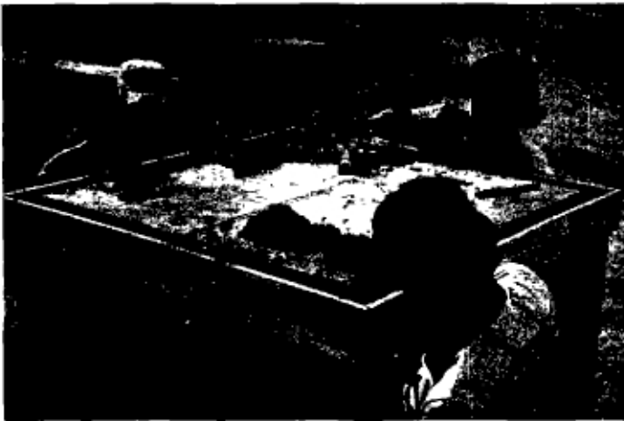
Illustrations 28 and 29: At least 12 hours after the corners are plastered. The corner boxing is removed and to correct any imperfections and cavities, a thin layer of 1 : 1 cement : sand mortar is plastered from the inside.
