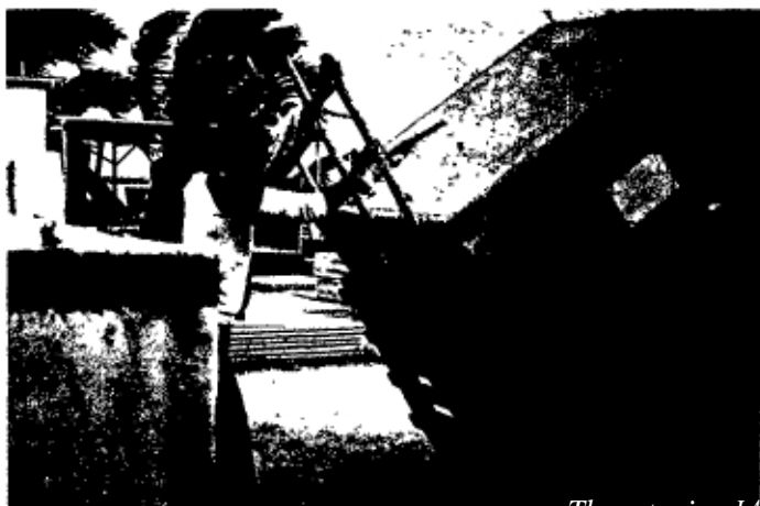
Illustrations 57 and 58: The tank is turned over after three days on a pallet for convenient transportation to the site of utilization.
