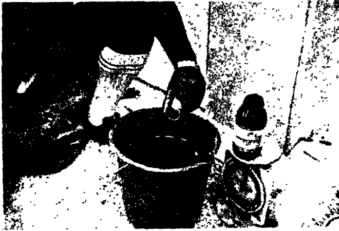
Illustration 3: If galvanized wires are used for reinforcement or fingering, an additive compound of hexavalent Chromium is required to be mixed with water for the preparation of the mortar.
