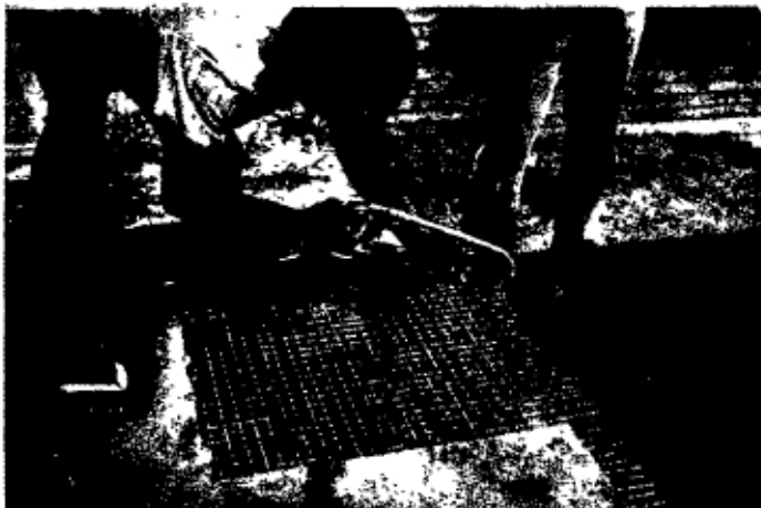
Illustration 47: For casting of the manhole panel, a blinder frame is constructed of size 60cm x 60cm (24" x 24") with saw slots on the bottom to match the wires.
