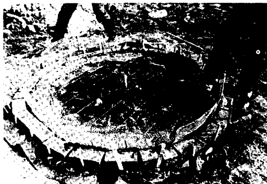
5.1 Note bricks acting as temporary formwork
