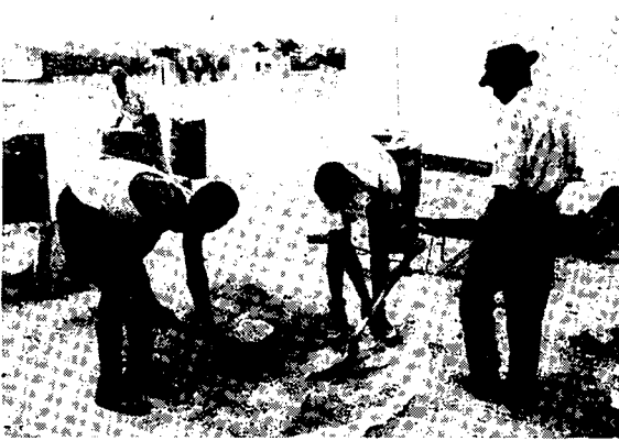
9.4 Mixing the mortar.
