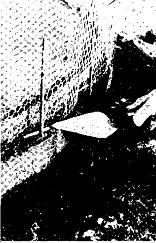
5.4 Bend up reinforcement
