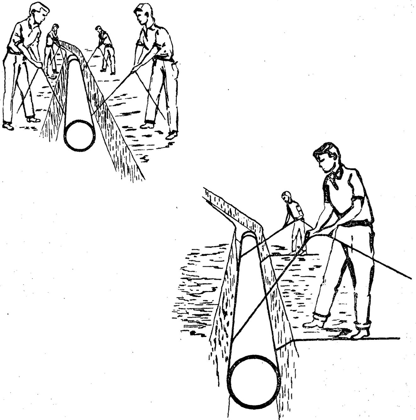
Fig. 19. Installation of pipes
