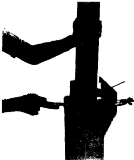
— When the endcap has reached the bottom of the well, lift the rising pipe up and push it down vigourously a few times until it does not move further down
