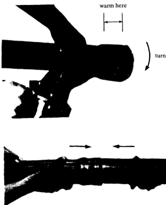
If there is any play, use the blow lamp to warm the expanded part (the socketed end) very carefully as shown in the picture. During warming, turn the pipe slowly.
