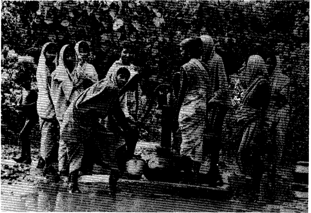
FIGURE 4-3 HAND PUMP WITH INADEQUATE DRAINAGE
