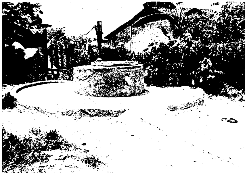
Nicaragua Site No. 21, located at Musuli (AID deep-well pump).
