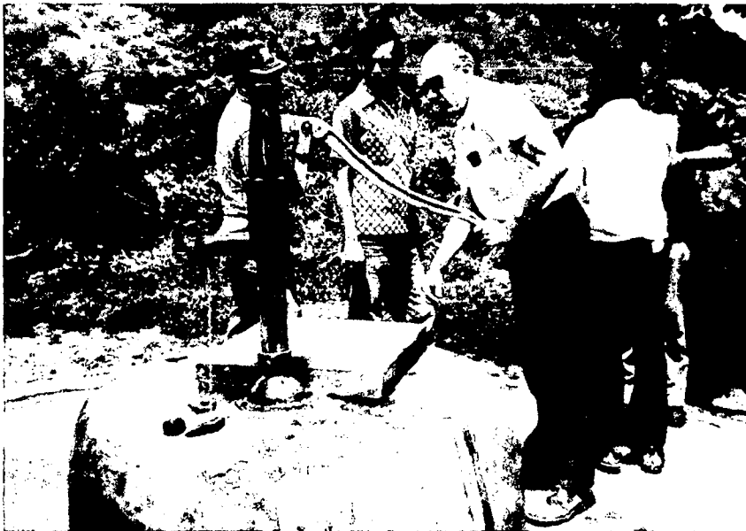
Nicaragua Site No. 19, located at Los Hatillos community plaza (AID deep-well pump).
