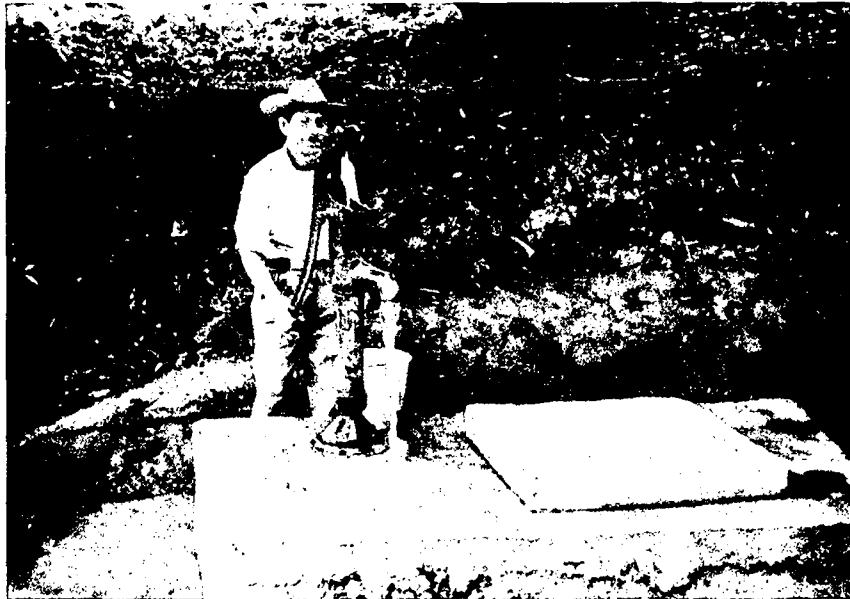
Nicaragua Site No. 27, located at Tomabu (AID shallow-well pump).
