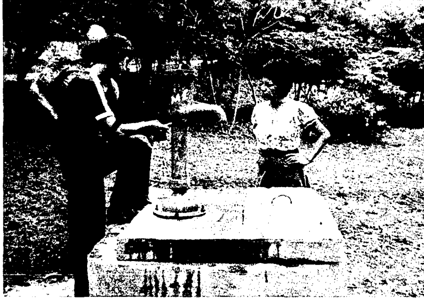
Site No. 19, located at Caimitalito de Nicoya (AID deep-well pump).
