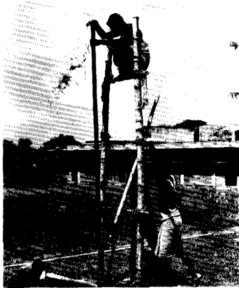
Figure 5.5 With very simple equipment, holes can be sunk to a depth of 50m in just a few hours (Photo Richard Cansdale)
