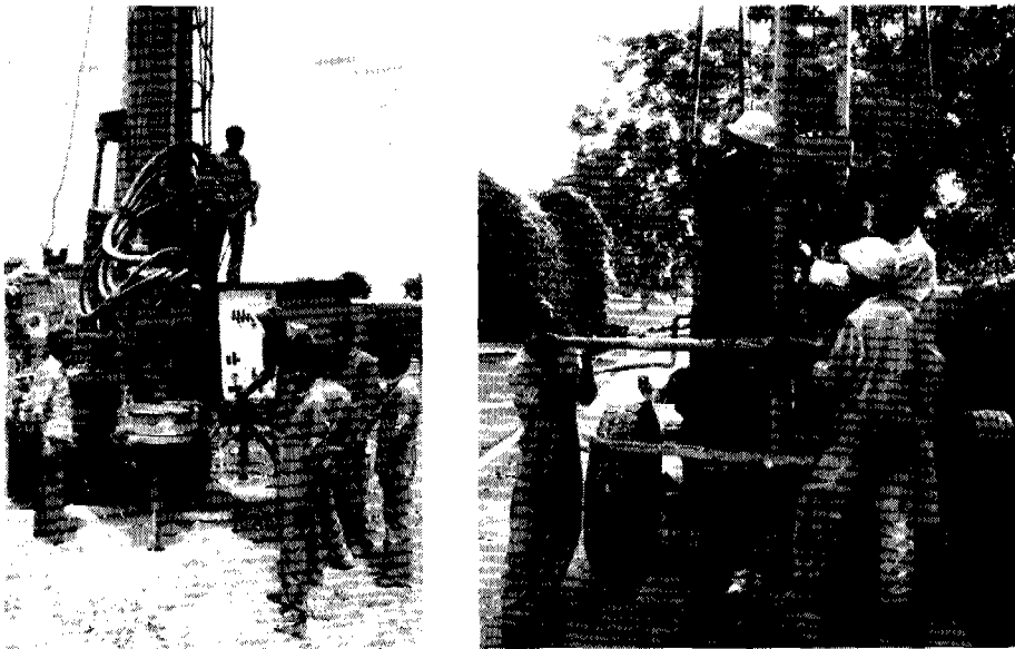
Figure 5.6 A cable-tool rig(left) and a high speed rotary rig (right)
