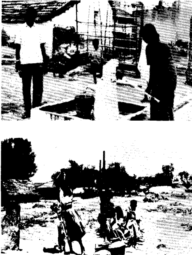
Figure 2.6 In the top picture, the pump handle is too low for comfortable operation, while in the lower picture, it is clearly too high. A height of about one metre above ground level has been found to suit most users. (Source: WHO/SEARO: 1976)
