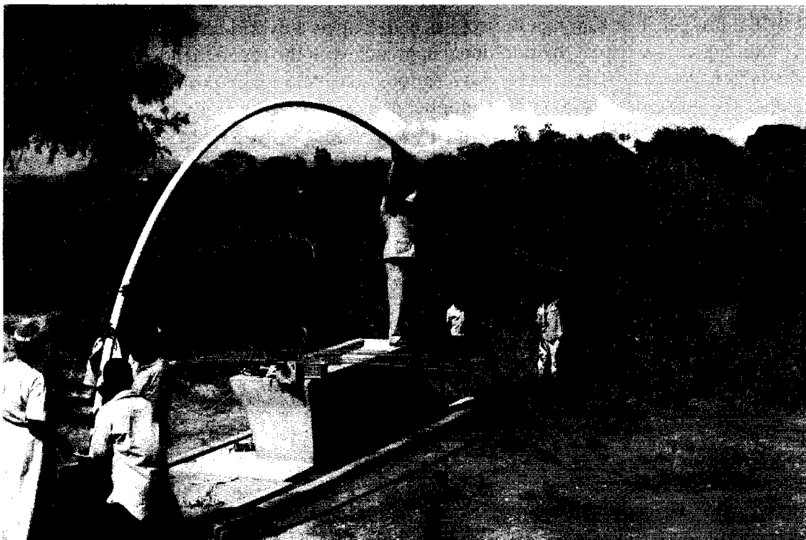
Figure 4: The community can be trusted - community members removing pumprods and rising main.
