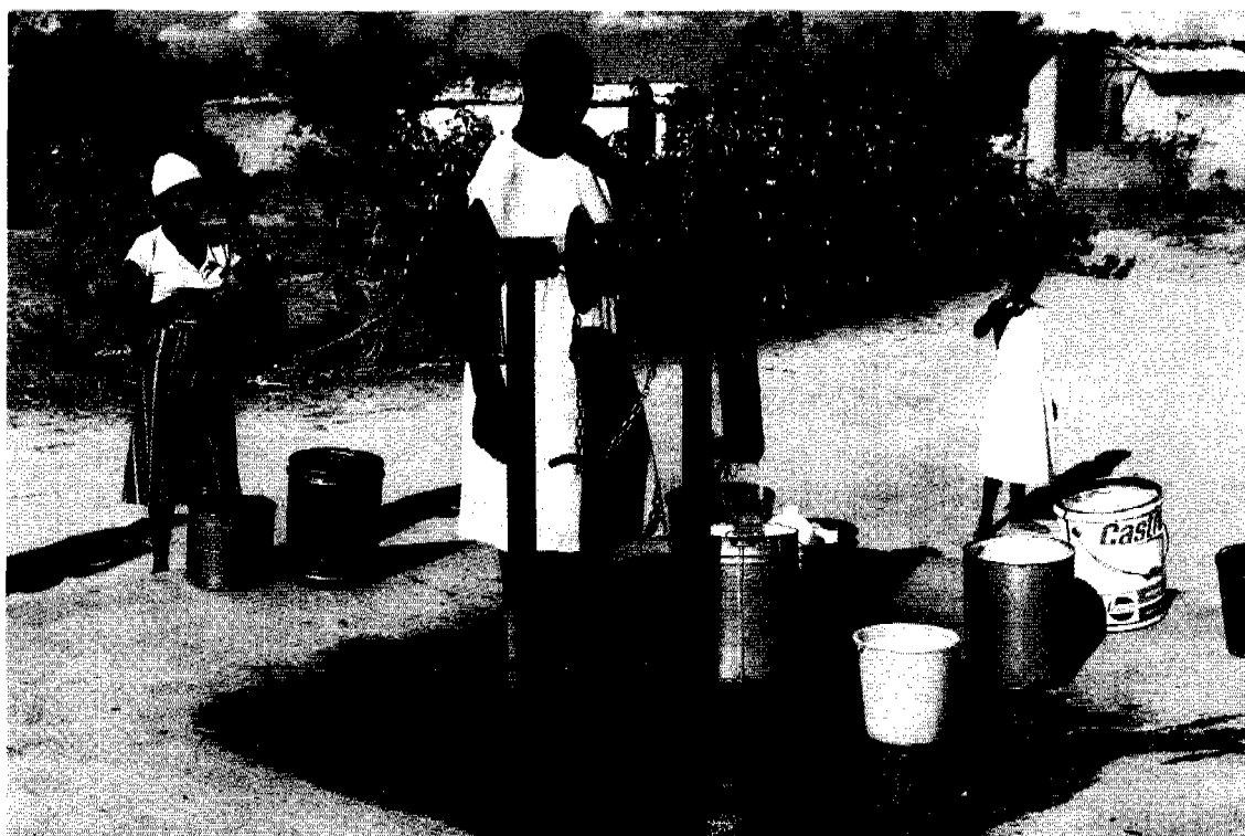
Figure A.2.1: The bucket pump in use in Zimbabwe.
