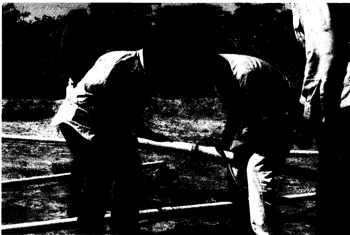
Figure 12: On-the-spot repairs to the rising main.
