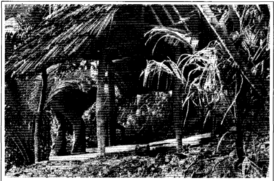
New toilets, like this one, under construction in Papua New Guinea, provide the best guarantee against diarrhea.
