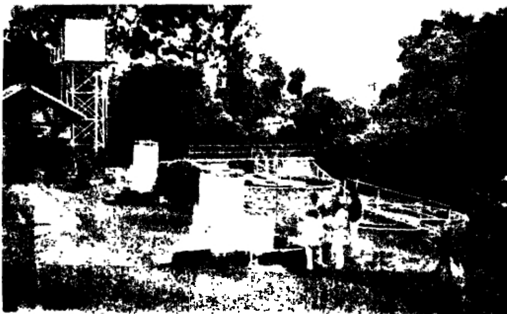
Ruiru town water supply. Filter backwash water tank left. Alum mixing and dosing units in the middle, circular horizontal settling basins are used.
