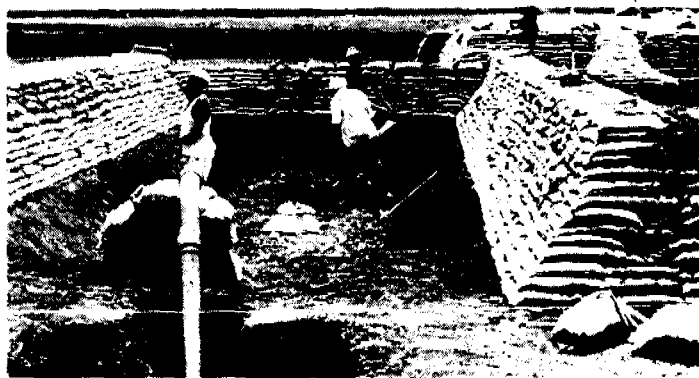
Fig. 10 Excavation of the HRF earth basin (picture by Swiss Disaster Relief Unit)
