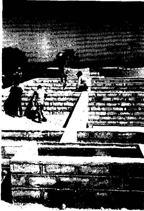
Fig. 8 HRF under construction at Kasote, Tanzania
