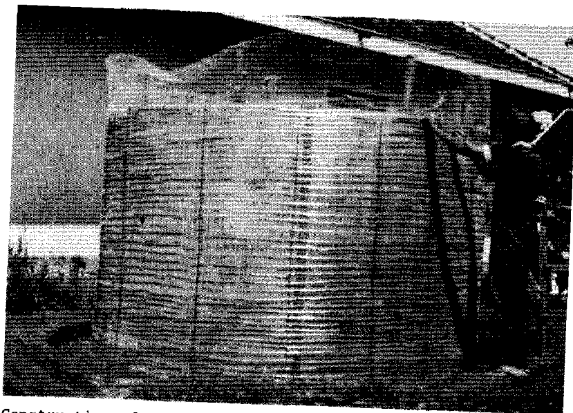
Construction of a ferro-cement water tank, Lombok, Indonesia.
