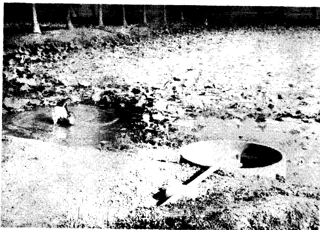
Raw water storage tank with intake well Pothunuru
