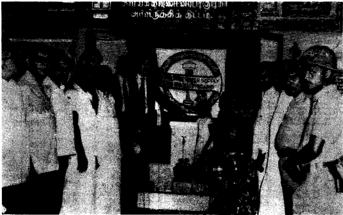
Formal commissioning of slow sand filtered water supply - Kamayagoundanpatti
