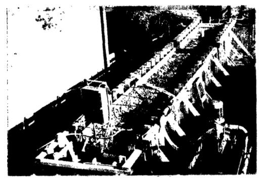
Figure 35. Filter media in place
