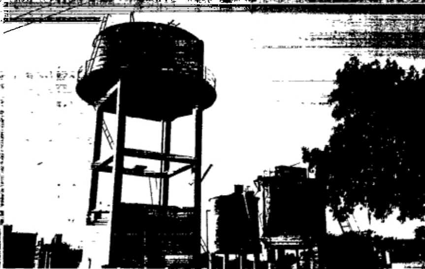
Plate 6. Fill-and-Draw Defluoridation Plant at Badarpur, Gujarat
