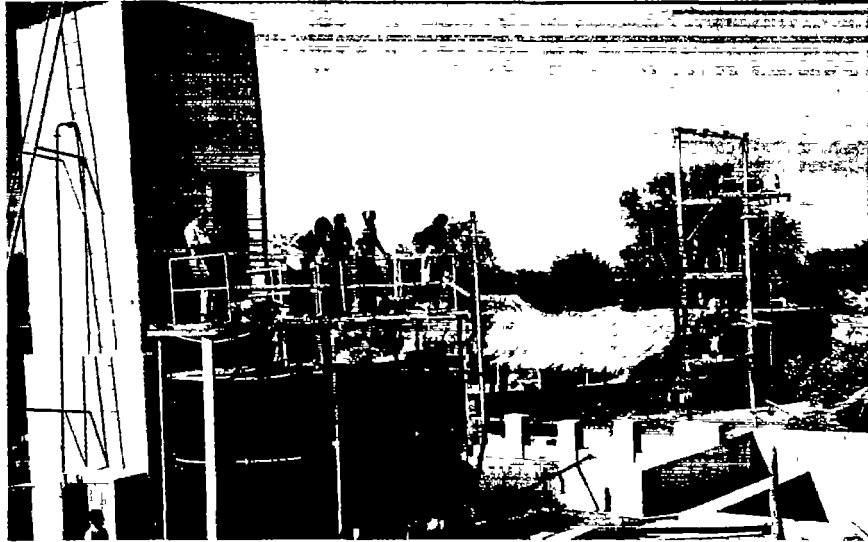
Plate 3. Fill-and-Draw Defluoridation Plant at Tartur, Andhra Pradesh
