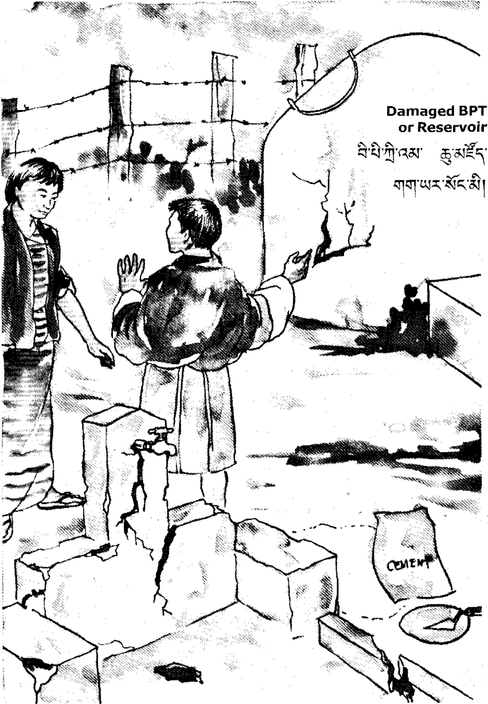
cracked Tapstand
