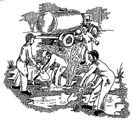
• When the main pipeline breaks the pumps must be stopped until it has been repaired.
