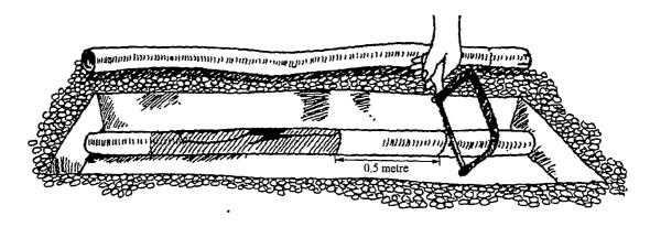
First cut the existing, pipe at least half a metre away from the damaged section using a hacksaw. Make the cut exactly square to the length of the pipe. Use a file to remove rough edges of the new cut. Do not let any pieces of polyethylene or dirt get into the pipe.
