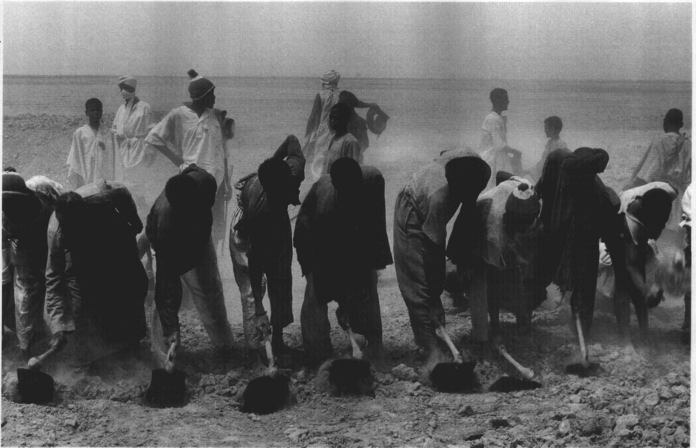
Working on an irrigation system in Mali.
