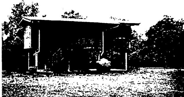
Figure 2. Obtaining rain water from the roof through a drain pipe.
