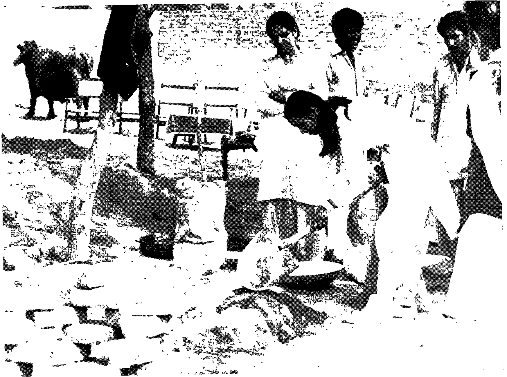
A lady promotor learns the proper technique for mixing cement.
