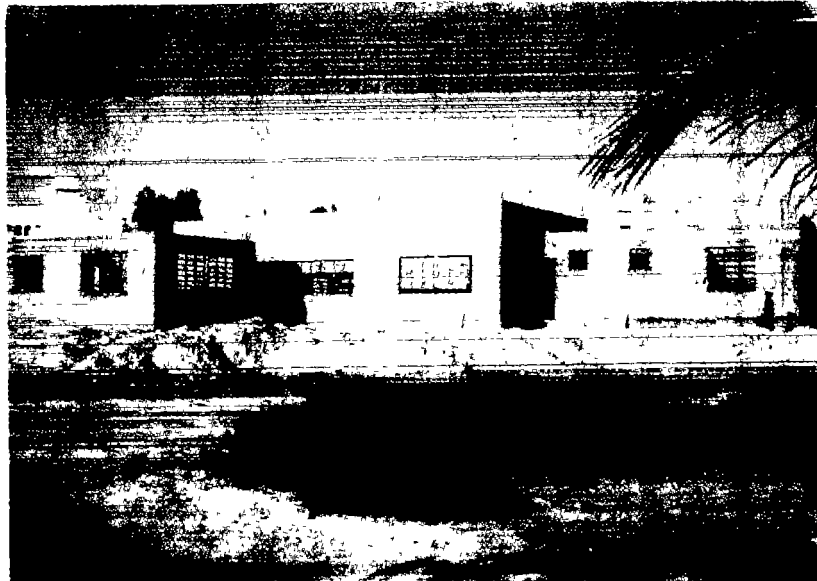
The RTI building under construction
