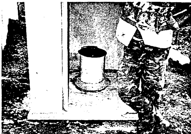
Fig. 14. The convertible riser installed.
