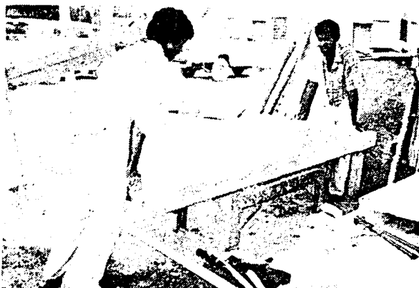
Fig. 4. Holding the mold while vibrating.
