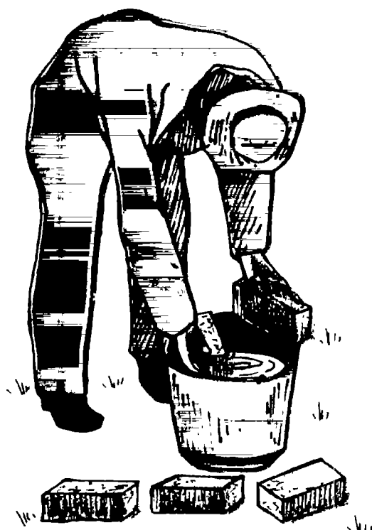
Soak the bricks before building
